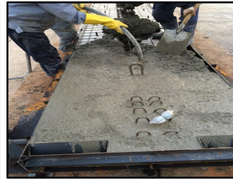
(4) Cast in Precast concrete
