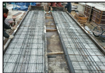
(6) Arrangement of re-bar in topping concrete
