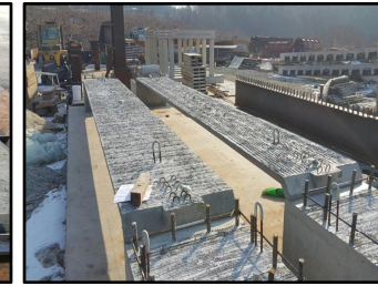
(5) Lift PC slabs on Beam
