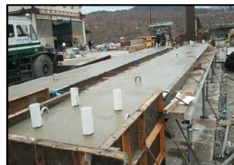
(7) Cast in topping concrete and curing
