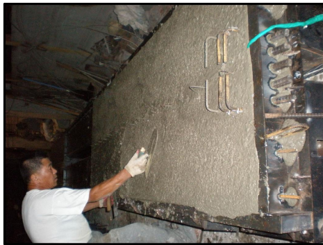
(4) Cast in Precast concrete
