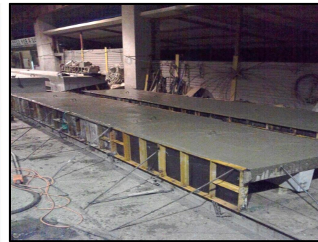
(6) Concrete curing
