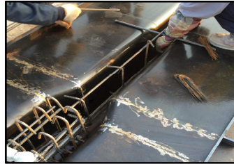
(2) Arrangement of re-bar
