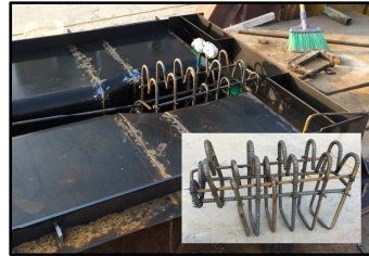
(1) Arrangement of re-bar in dapped end
