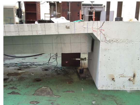
(ii) Completion stage
