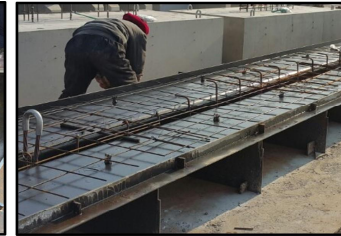
(2) Arrangement of re-bar
