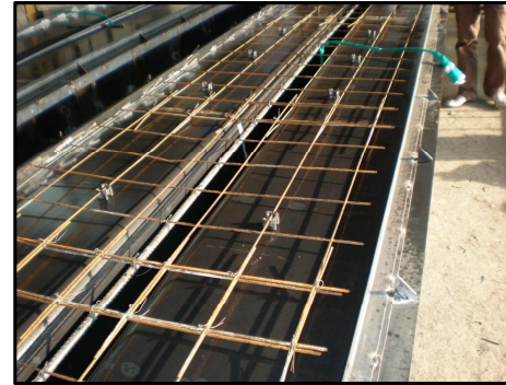
(3) Arrangement of re-bar
