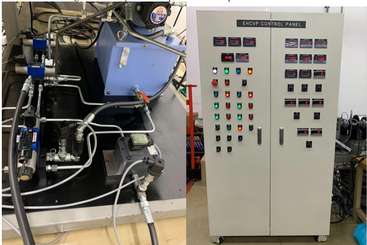
Fig. 3-7 Hydraulic system and control box in experiment test bench.
