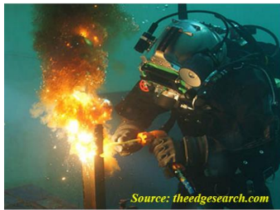
Ignition and explosions
