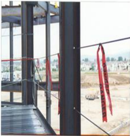
Specify holes in columns at 21 and 42 inches above the floor slab. This design feature makes it easy to install cable or wire perimeter cables.
