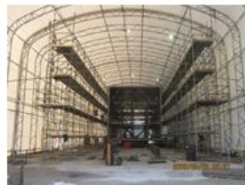
Figure 2 – This photo shows work inside the tent.
