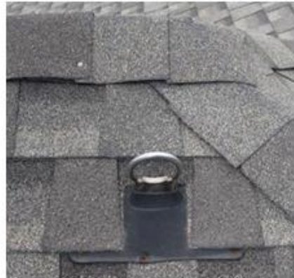
Figure 2 Residential roofing has a high incidence of falls. Installing residential roof anchors provides a place for workers to tie off.
