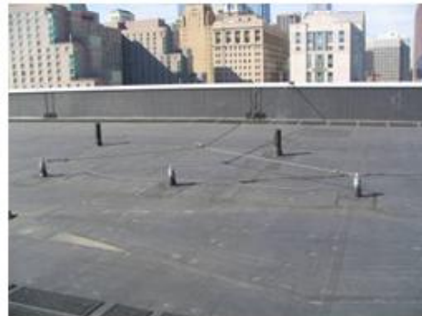
This photo shows permanent roof anchors. Specifying multiple roof anchors will provide convenient tie off points when working near the edge of the roof.
