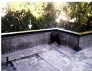
This photo shows a parapet wall around the roof edge.
