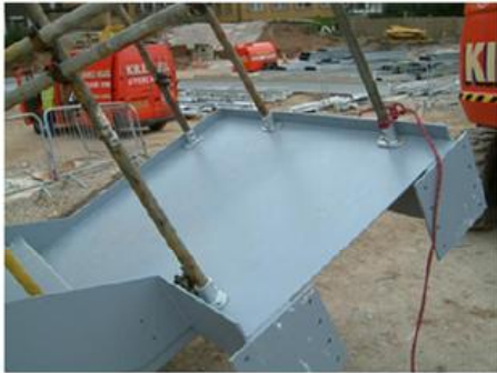
Temp. stair handrails installed at ground level (Same holes were later used for the permanent handrail)
