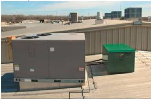
This photo shows equipment located on a roof. Positioning equipment at least 15 feet back from the roof edge will reduce the risk of falling when installing and servicing the equipment.
