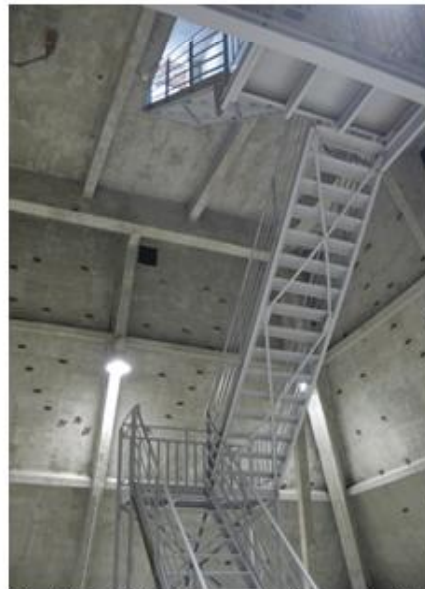
Fixed industrial stairs can also be specified to access an a work platform, mezzanine, upper level, or a roof. Alternating tread devices can be specified if there is limited space.
