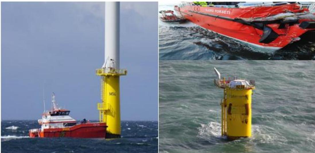
Figure 6.1 Collision damaged of offshore wind turbine platform column [6-1 & 2]
