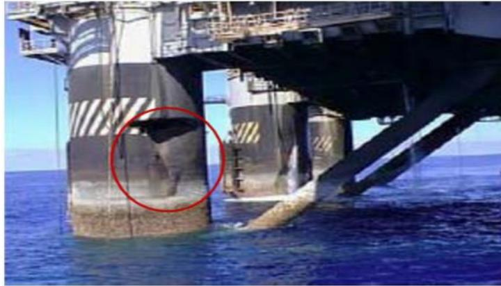
Figure 6.2 Collision damaged of offshore platform column [6-4]
