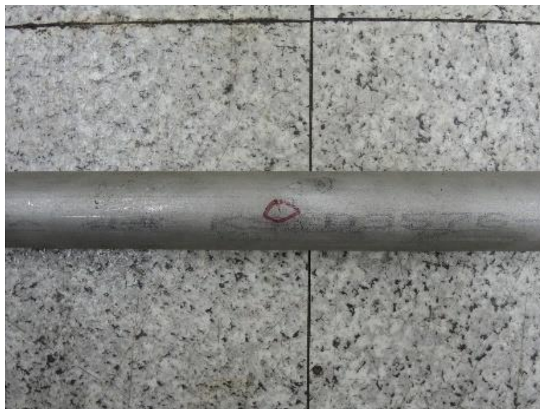
Figure 7.2 A simulated leak orifice of the pipe.
