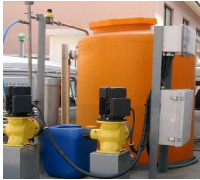
[Fig 23] Spray test system used in field experiments
