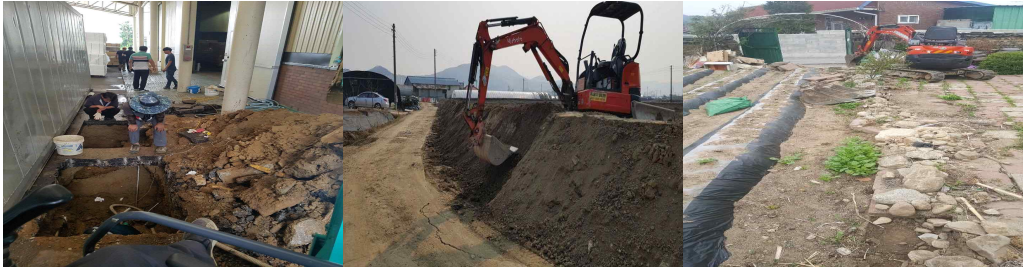
Fig. 2 Excavation work using field robot
