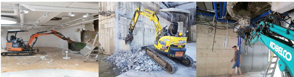
Fig. 4 Demolition work using field robot
